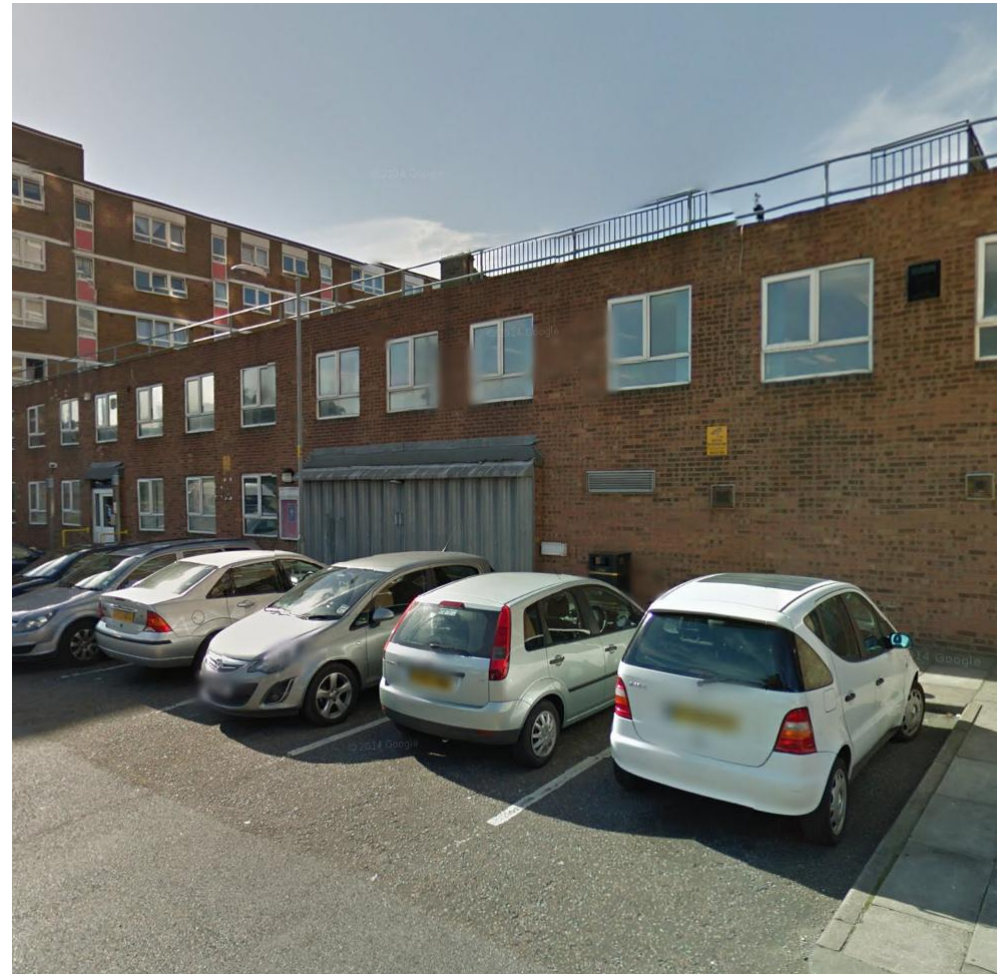
Photograph of Site
